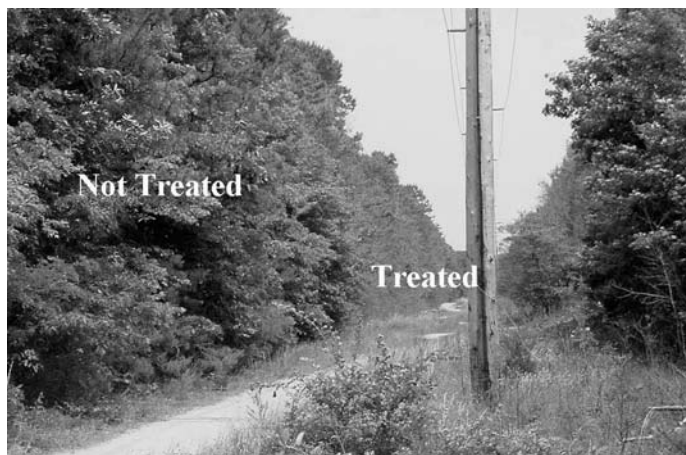
Here are the one-year results of ULV side trimming on the Conectiv 69kV transmission right-of-way in New Jersey. The green trees are low-growing species that were left untreated. Use of the ULV Thinvert application system provides a higher percentage of control, reduced understory damage of desirable vegetation, and higher crew productivity.
